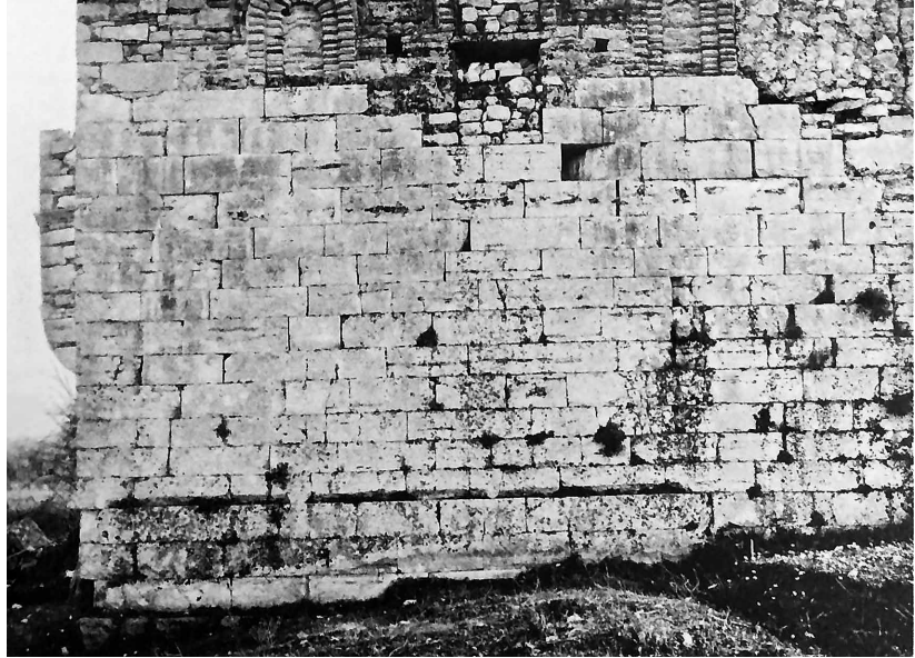
Figure 39. Isodomic ashlar masonry of the fortification tower and wall at the Church of Panayia Nerantzicha, Corfu (Korkyra). Korkyra 1, pl. 1; courtesy Verlag Gebr. Mann, Berlin
